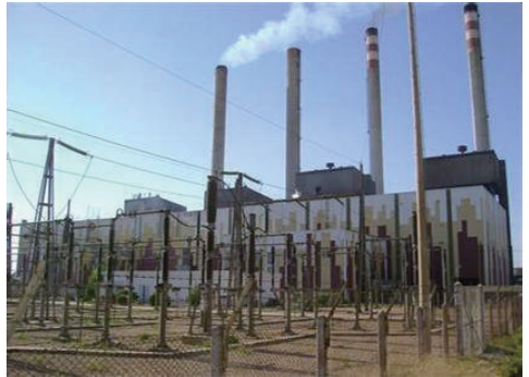
Meharkeh Power Station ,Syria
