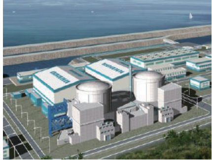
Ling Ao Nuclear Power Station
