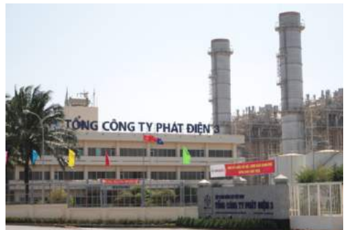
EVN GENCO 3 - Phu My Thermal power Company Phu My 1 IZ, Tan Thanh, BRVT, Viet Nam
