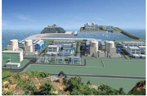
Fujian Ningde nuclear power plant
