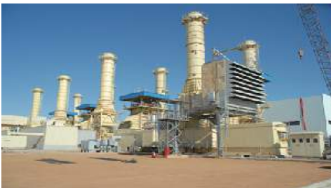
Cam Pha Coal-fired Thermal Power Plant, Vietnam
